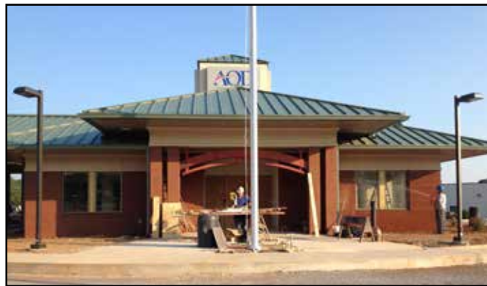
New AODFCU Jacksonville Office
